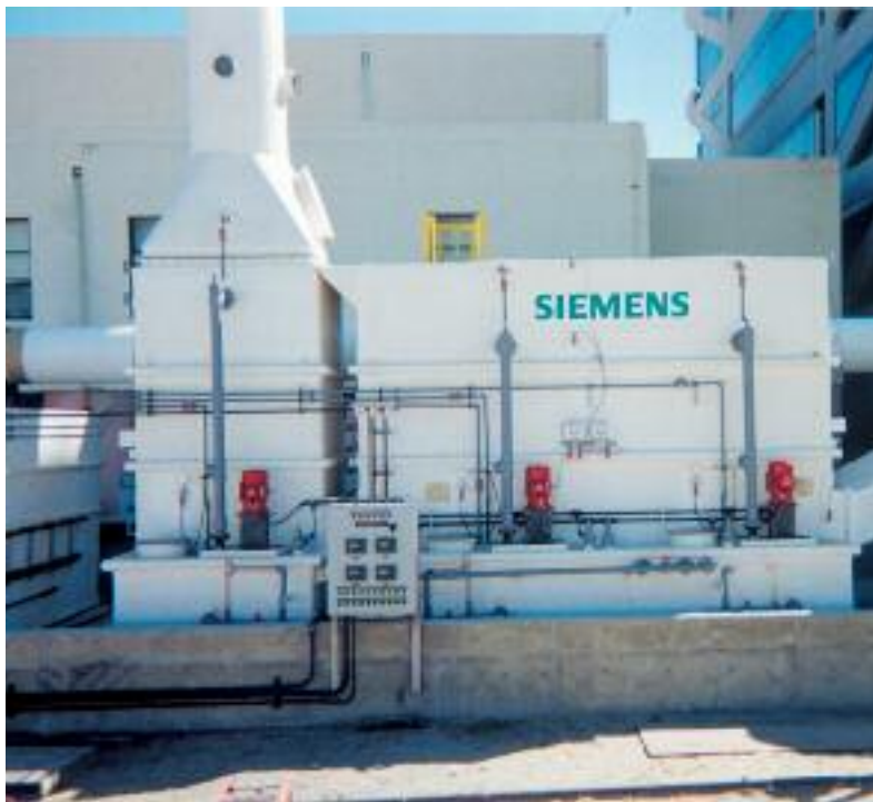
The LO/PRO® scrubber is a high efficiency "wet chemical" scrubber, all in a small footprint.
