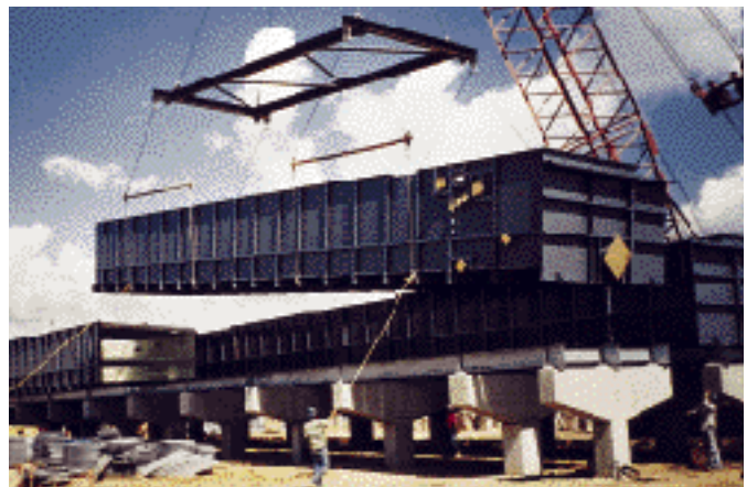
Four, 16-foot (4.88 meter) wide by 160-foot (48.76 meter) long API oil/water separators were shop fabricated and finish painted before shipment.
