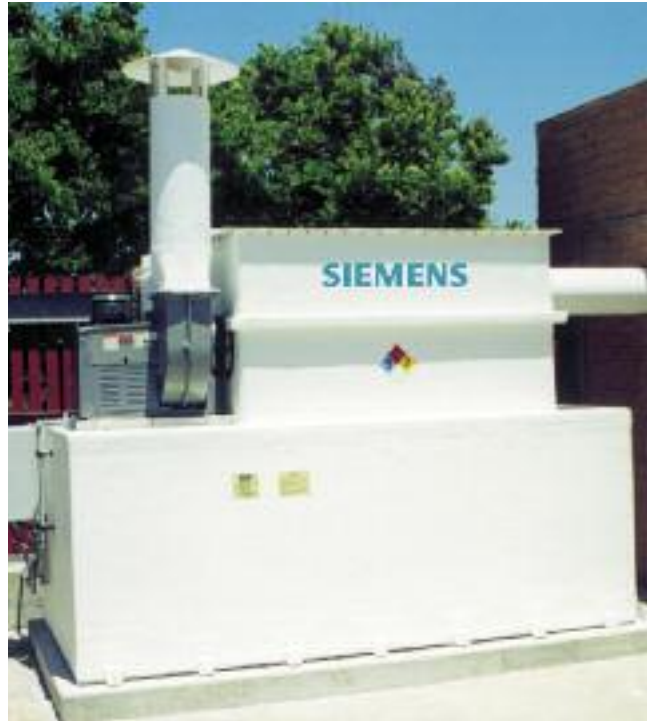
Emergency vapor scrubber systems prevent potentially dangerous gas release.
